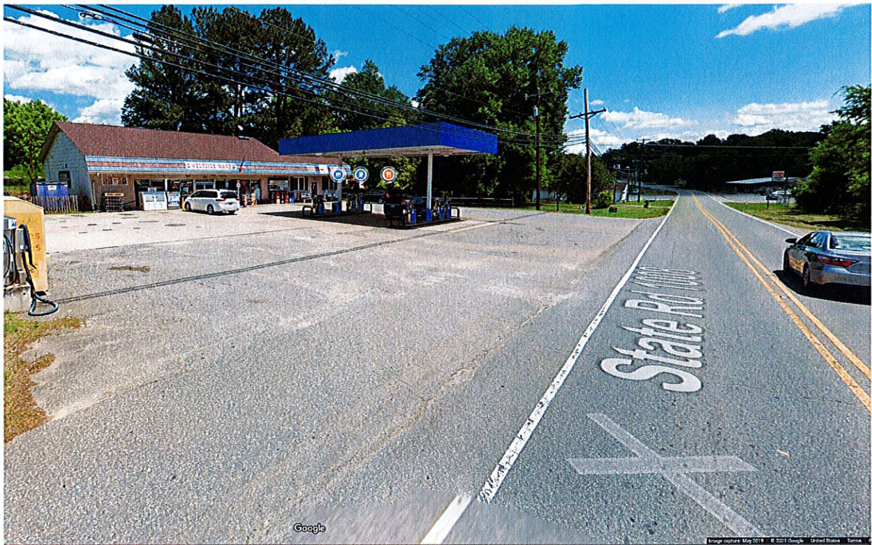
Canopy Prior to Wind Damage 2020
