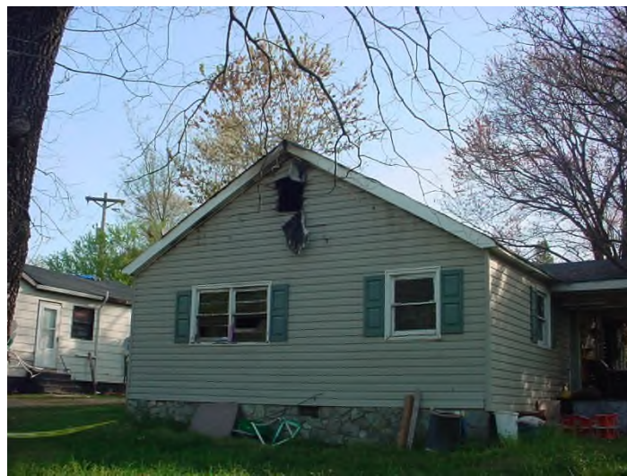
Left side view / Gable vent removed Smoke / fire damage
