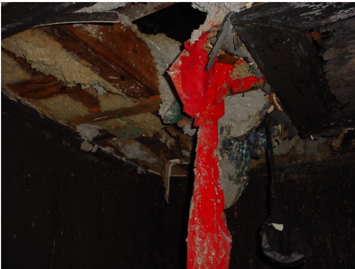
Ceiling material loose, missing, Severely fire, smoke and water damaged
