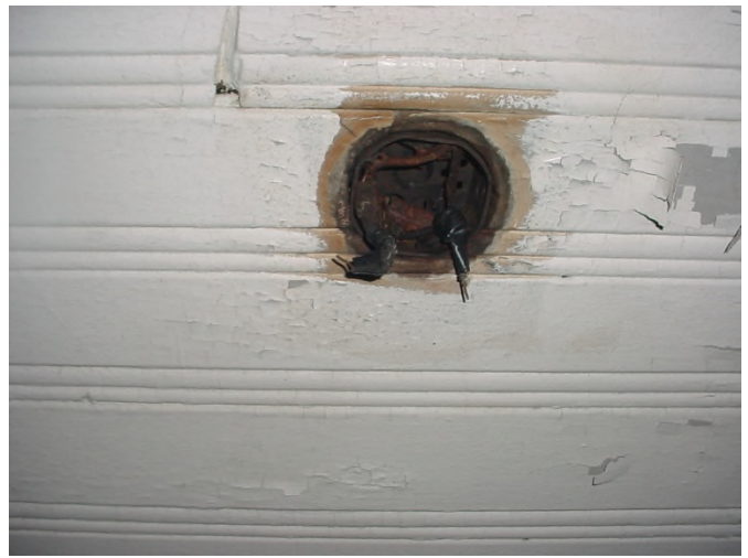
Ceiling light fixture missing / wiring exposed
