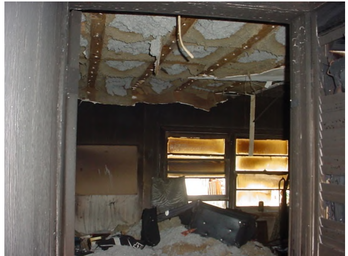
Ceiling material loose, missing, Severely fire, smoke and water damaged
