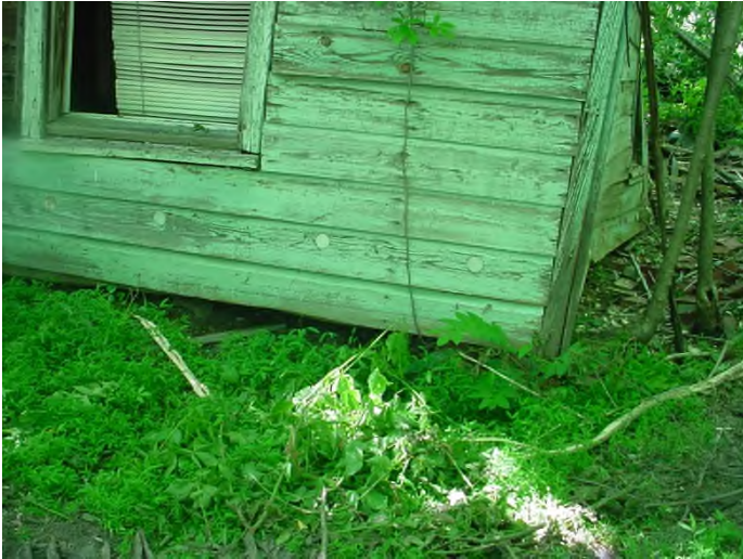
Windows defective / Wall System collapsed
