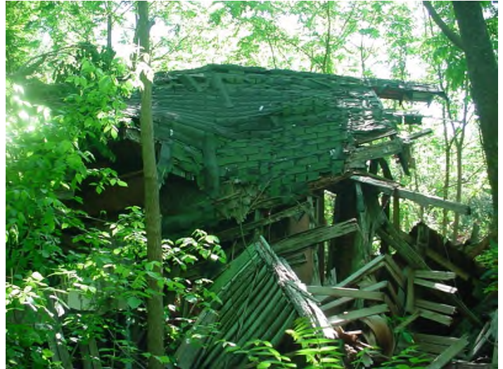
Roof system collapsed / Wall System Collapsed
