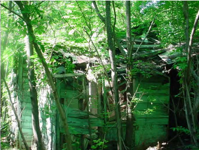
Windows defective / Wall System collapsed
