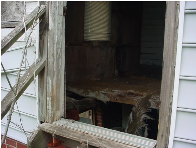
Holes in floors / sills and joists deteriorated
