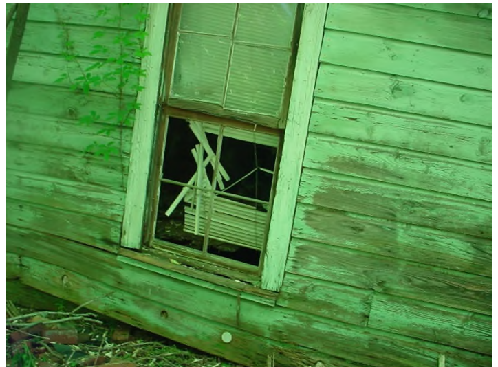
Roof system collapsed / Holes in exterior walls / Windows broken (Not weathertight)
