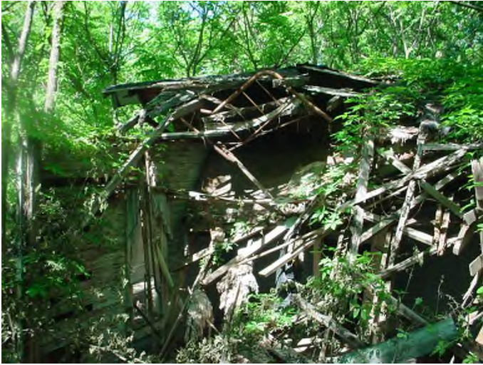
Roof system and wall system collapsed
