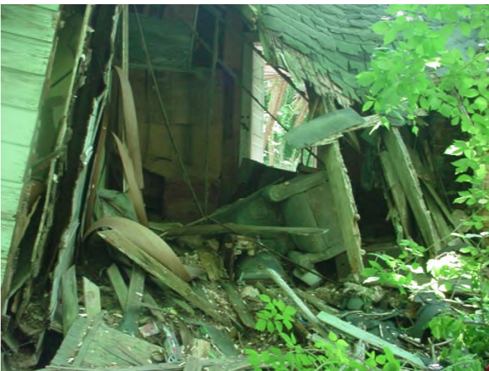
Roof system collapsed / Holes in exterior walls / Windows broken (Not weathertight)
