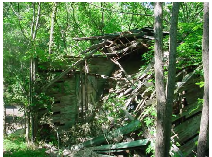
Roof system collapsed / Holes in exterior walls
