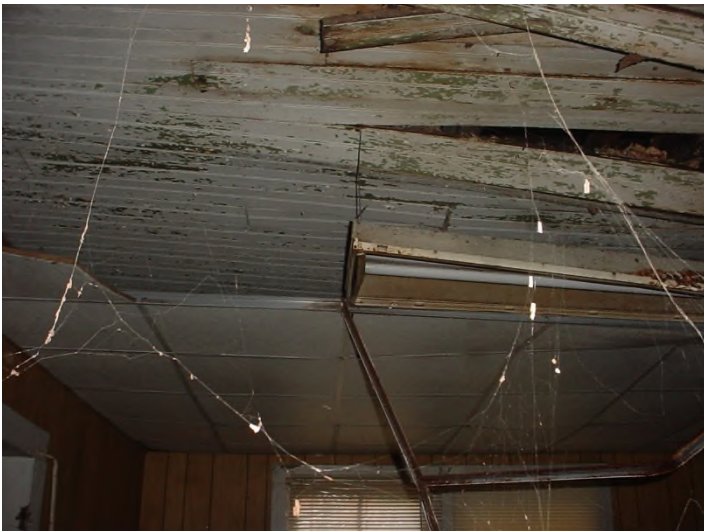
Holes in ceilings / Mold and mildew at ceilings
