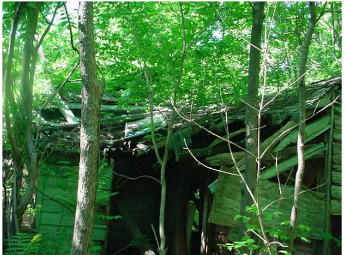
Roof system collapsed / Holes in exterior walls
