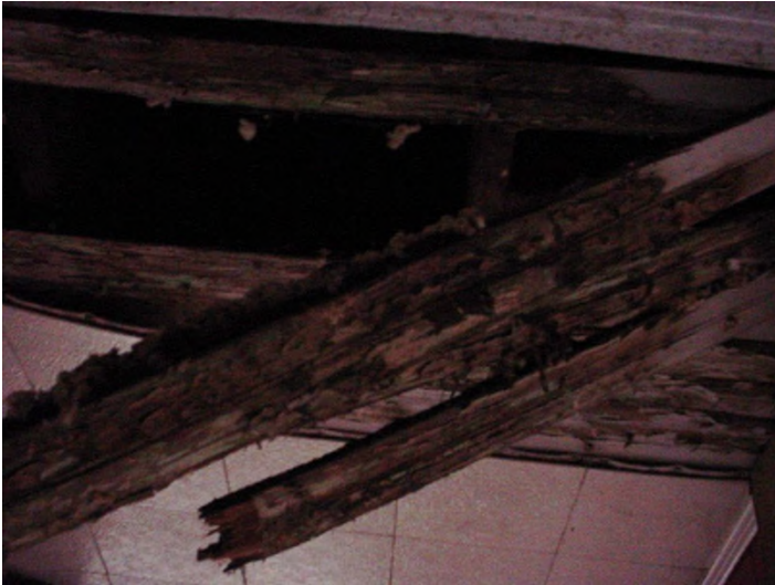
Holes in ceilings / joists and rafters deteriorated / Insulation loose and water damaged
