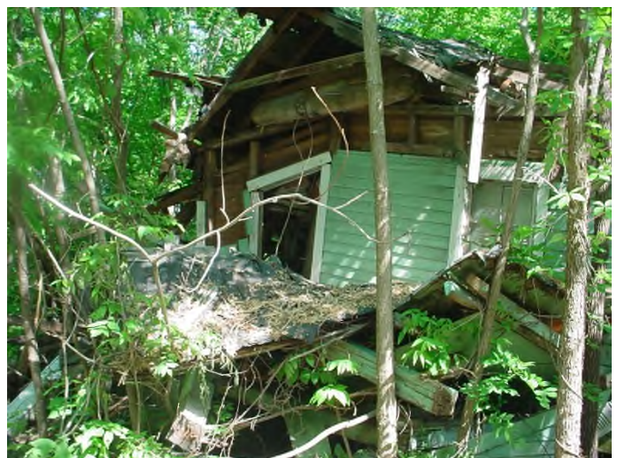
Roof system and wall system collapsed
