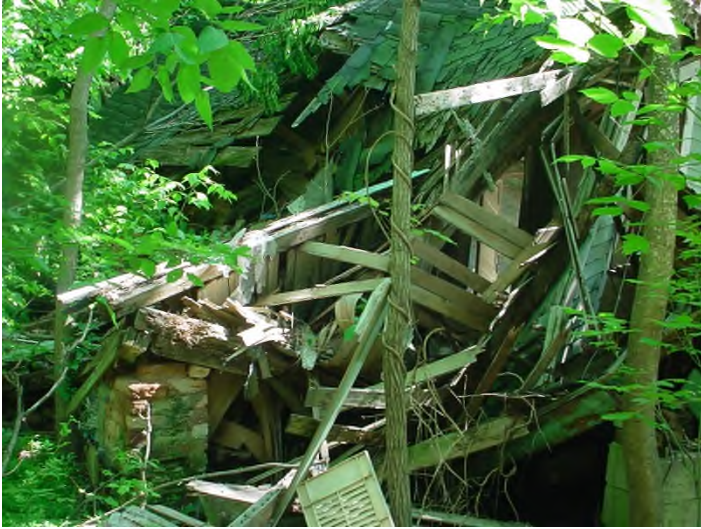
Roof system collapsed / Wall System Collapsed
