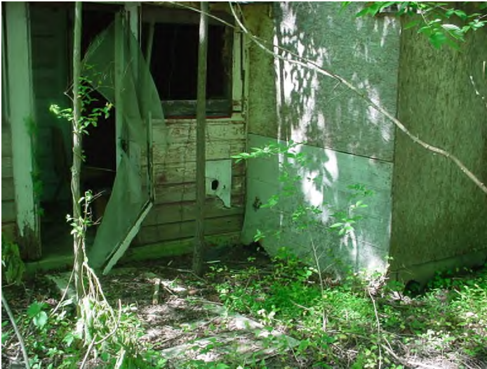
Screen porch defective Screen torn / Framing damaged
