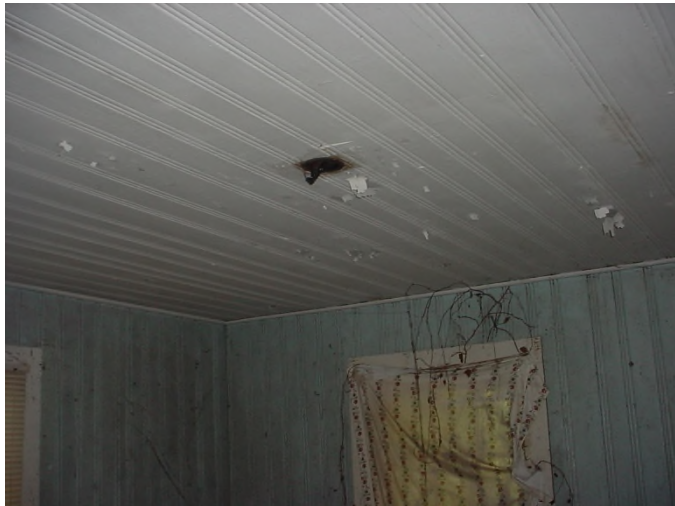
Ceiling light fixture missing / wiring exposed
