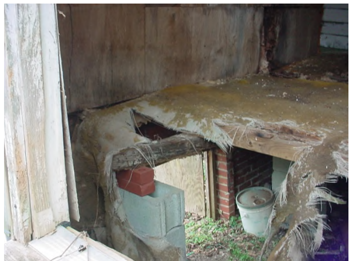
Holes in floors / sills and joists deteriorated
