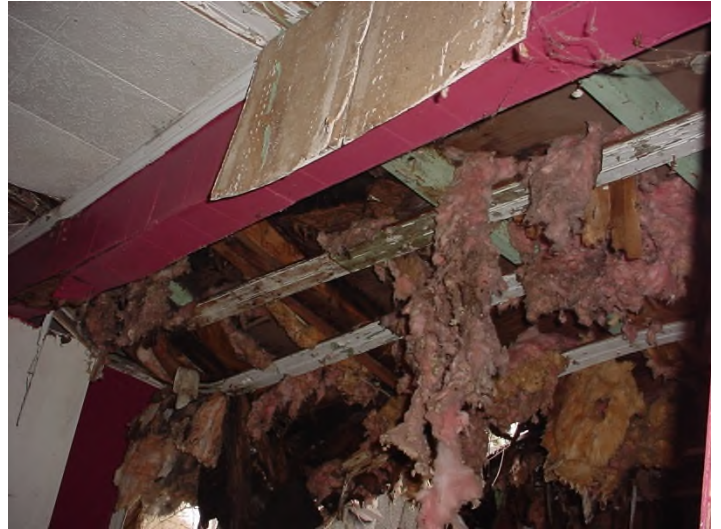
Holes in ceilings / joists and rafters deteriorated / Insulation loose and water damaged
