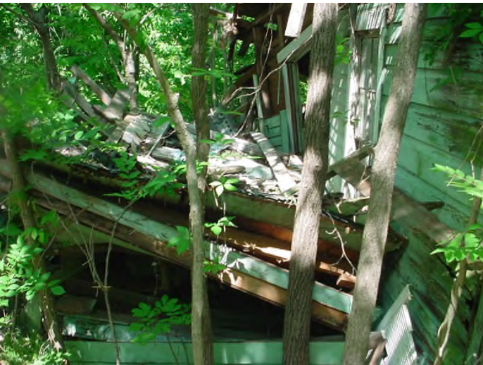
Roof system and wall system collapsed
