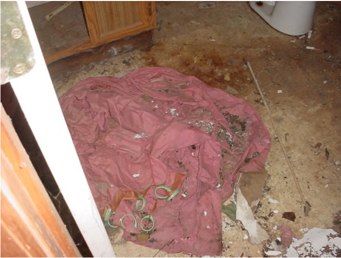
Bath flooring unsanitary / Trash and debris throughout
