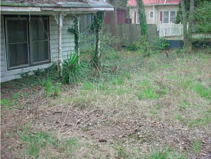
Grass and weeds overgrown
