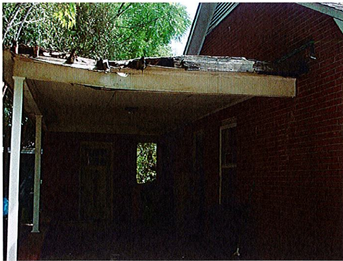
Carport roof / ceiling deteriorated
