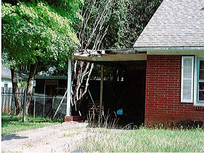
Carport roof / ceiling deteriorated
