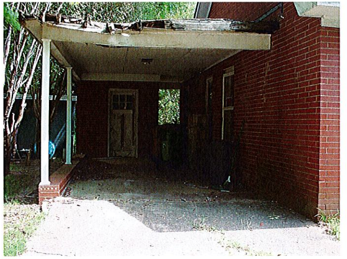
Carport roof / ceiling deteriorated
