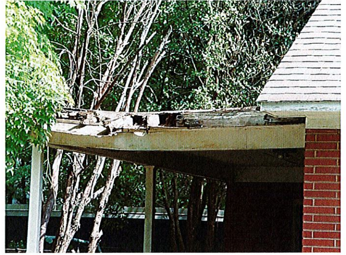
Carport roof / ceiling deteriorated
