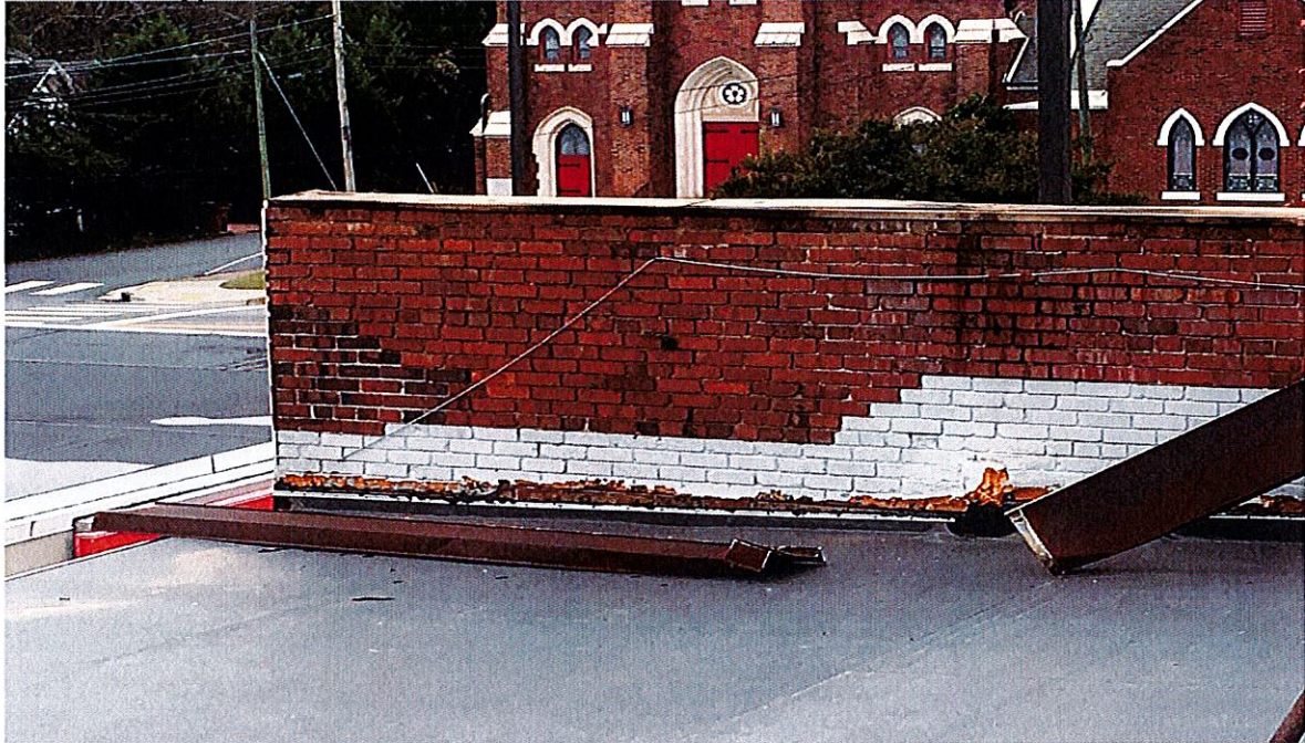
Photo 3 – Typical Condition of Lower Roof. Failed base flashings. Missing metal coping.
