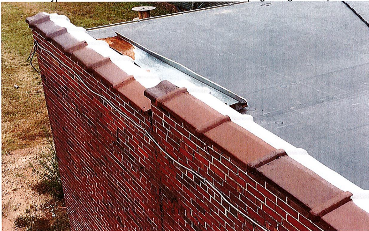
Photo 4 – Typical Condition of Lower Roof. Terra cotta coping is in good shape.
