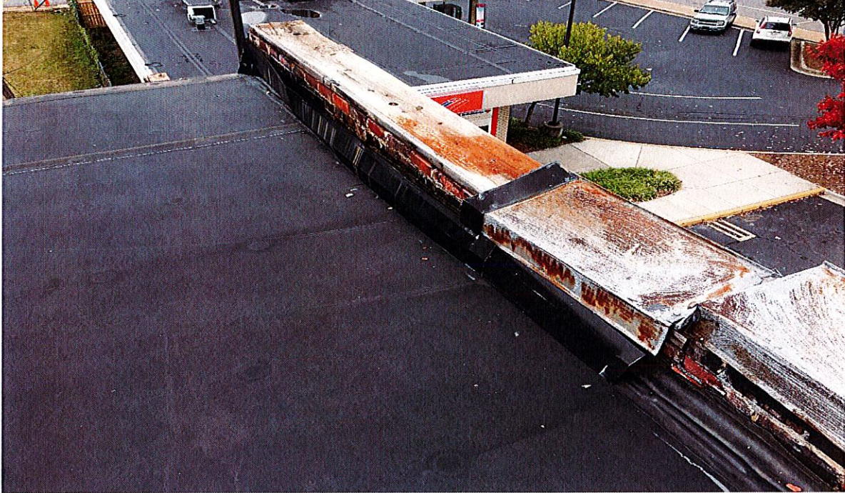
Photo 1 – Typical Condition of Upper Roof. Failed base flashings. Failed metal coping.
